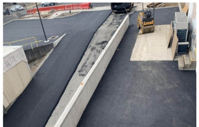
Parking Lot Paving
